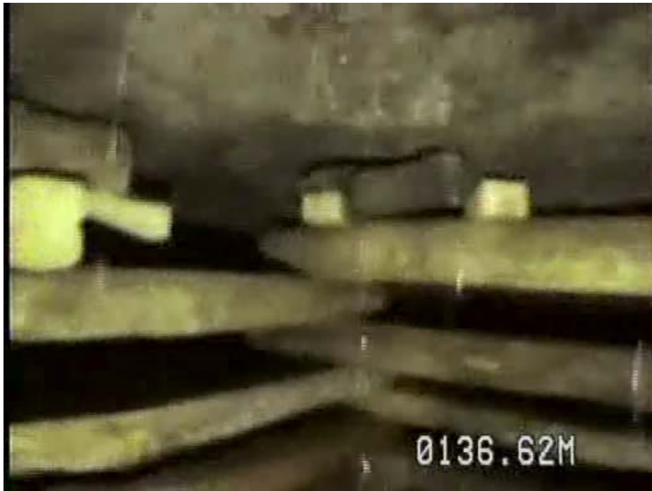
Figure 4.25. Another view of M-8 cribbing
