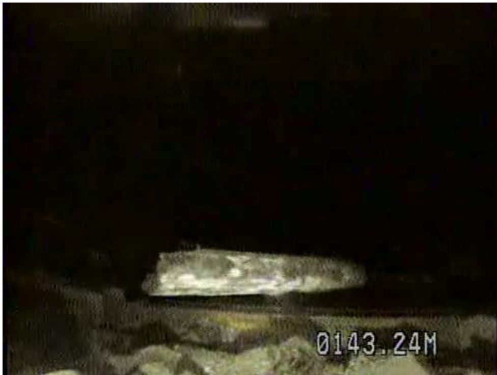
Figure 4.20. C-24 materials on the floor
