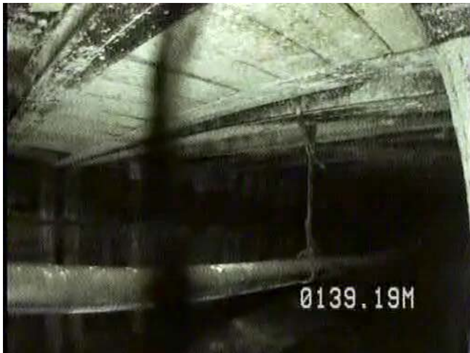
Figure 4.18. De-gas 7 Shows rehabilitate structure still intact
