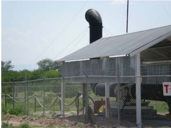
Figure 3.1 Bleeder borehole fan.
