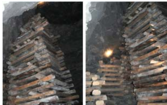
Figure 2.5 Cribbing to support caved area.
