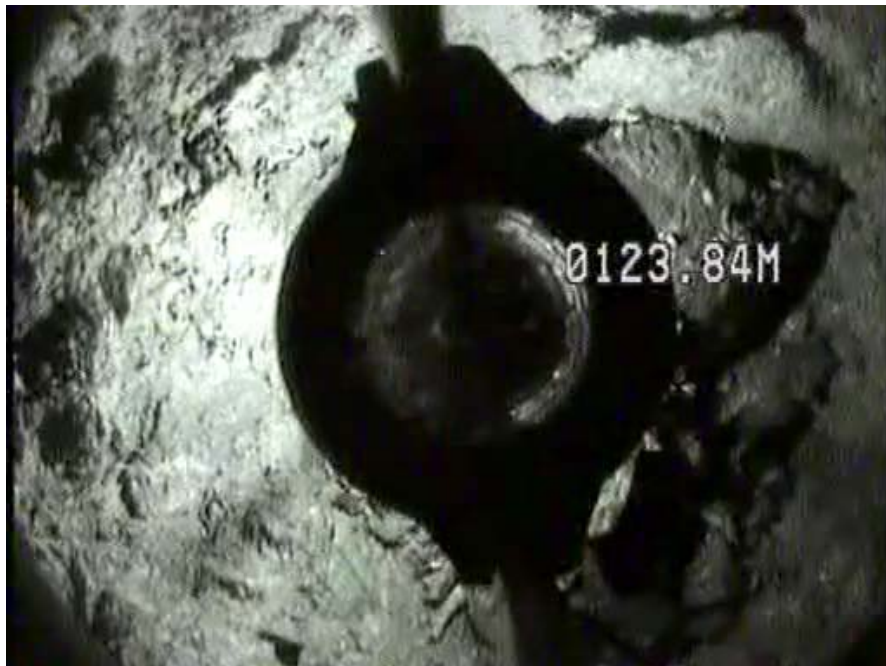
Figure 4.22. C-6 Obstructed at 124 Meters
