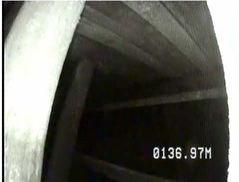
Figure 4.17 De-gas 5 Hole intact support structure
