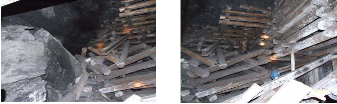
Figure 2.6 Collapsed cribbing at cross-cut 13.
