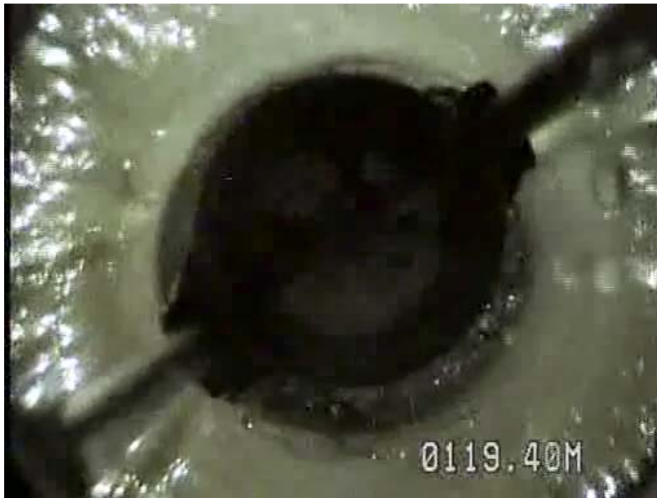
Figure 4.8b. C-10 Blockage as seen from 119.4 meters
