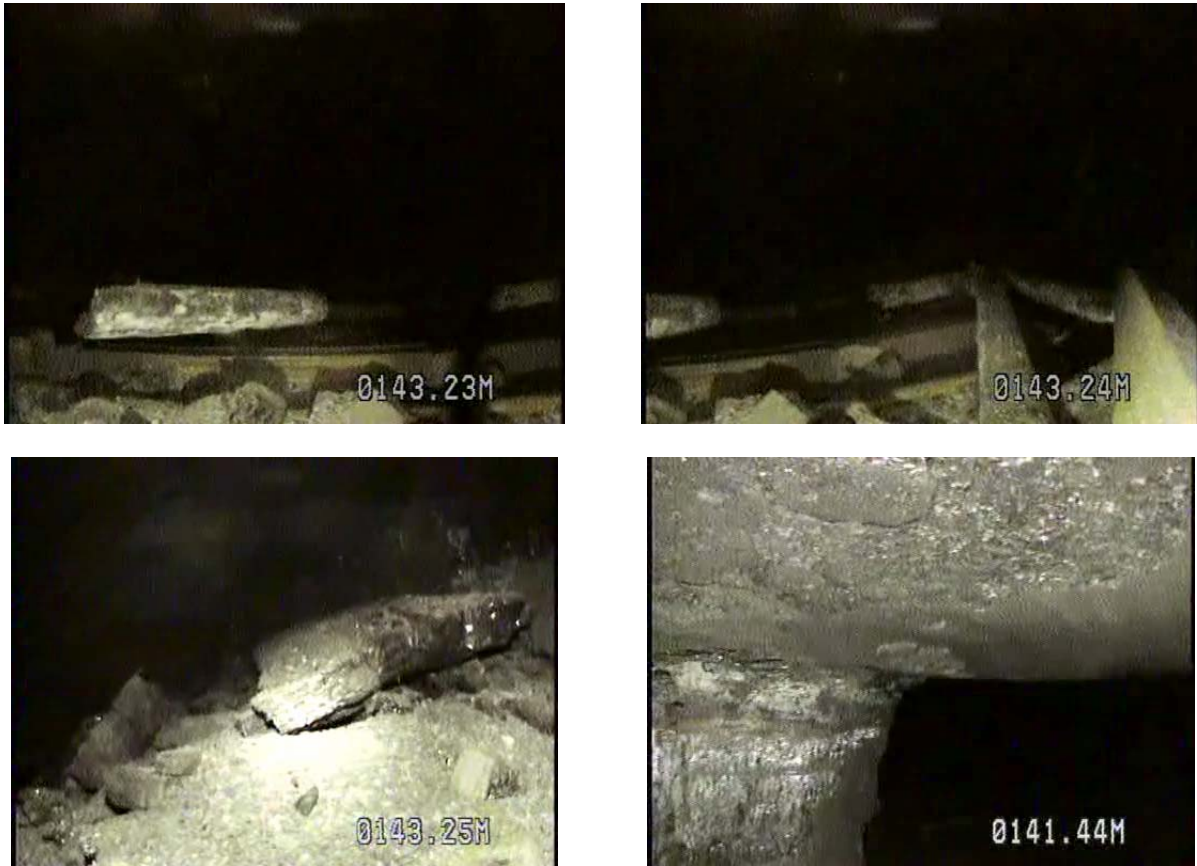
Figure 2.15 Snapshot from borehole C-24
