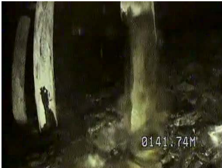
Figure 4.16. Borehole C-20 support posts still standing
