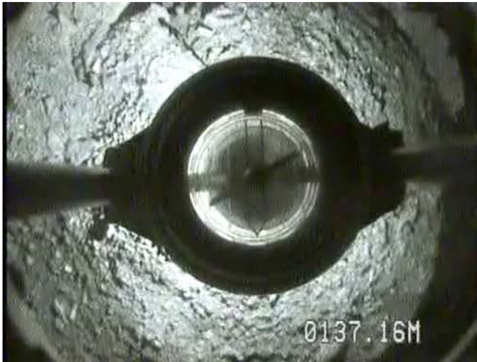
Figure 4.11. C-26 Obstructed borehole at 137 Meters
