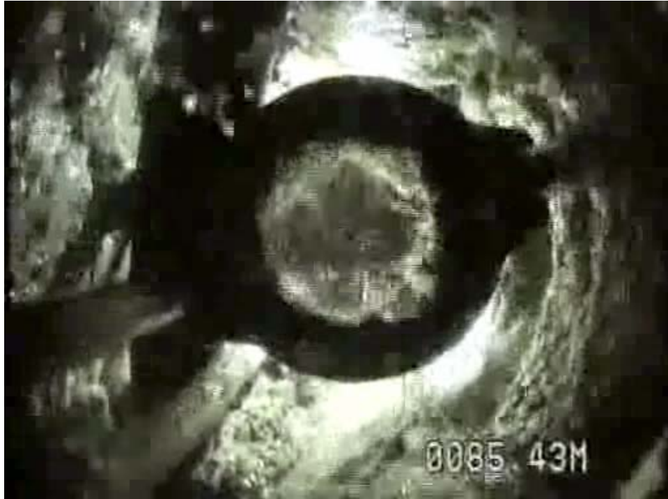
Figure 4.23. Running water in Obstructed M-7 at 85 meters
