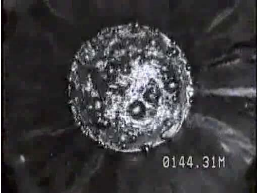
Figure 4.9. Water and gas bubbling at C-11
