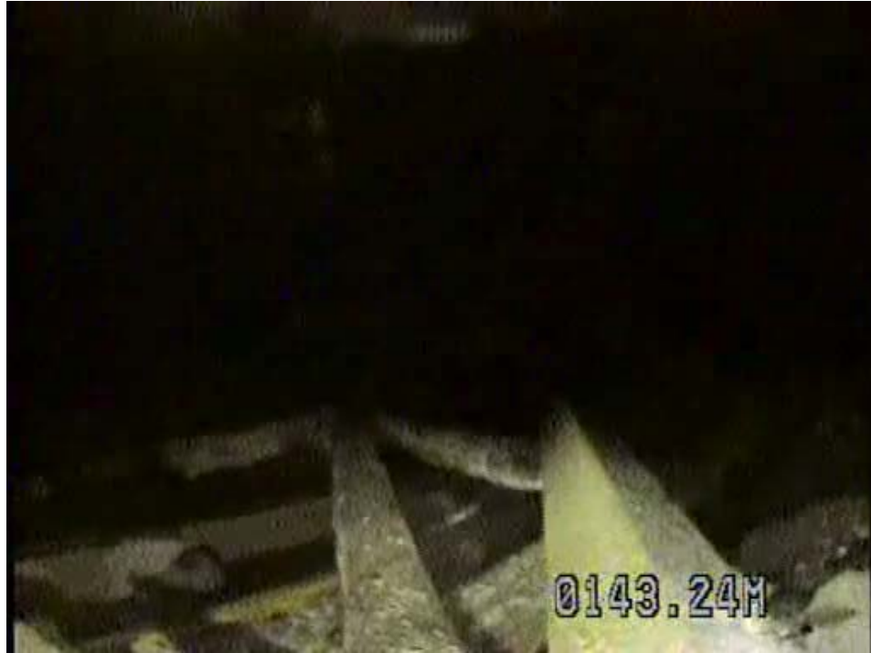
Figure 4.19. C-24 materials on the floor
