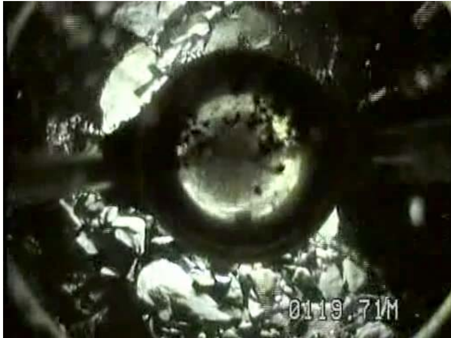
Figure 4.8a. Debris Blockage in C-10 as seen from 119.71 meters
