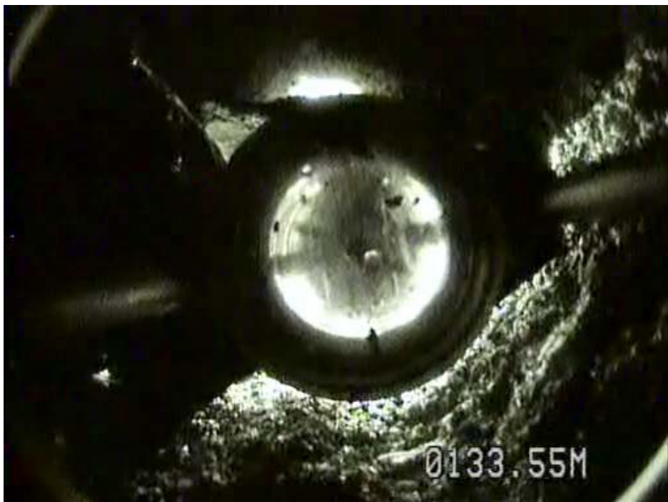
Figure 4.10. C-23 Obstructed borehole at 133 meters
