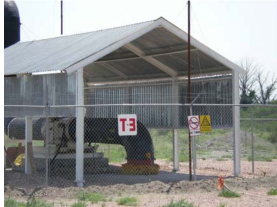
Figure 3.2 Bleeder borehole fan.
